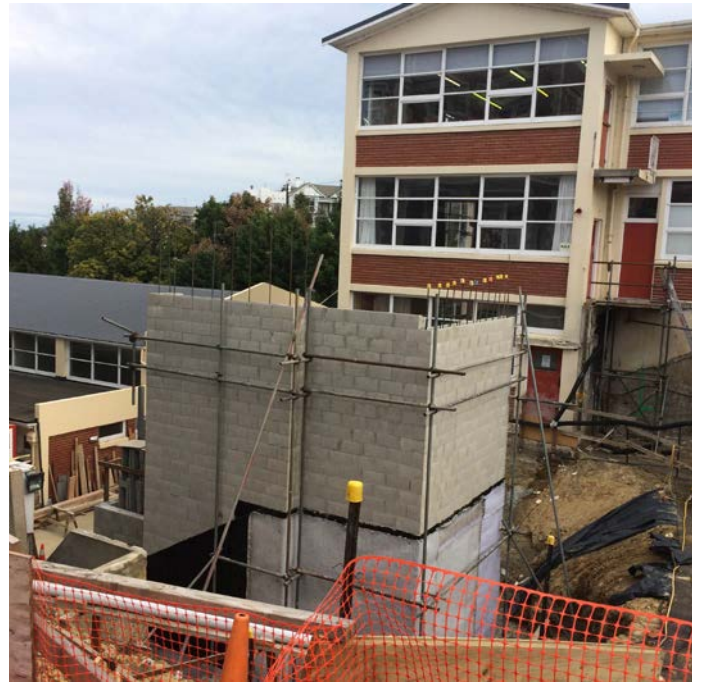
Development of the new access tower and music suite, April 2015.
